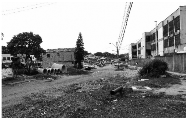
Figure 4. Tronco Avenue roadworks next to the roundabout, November 2017.
